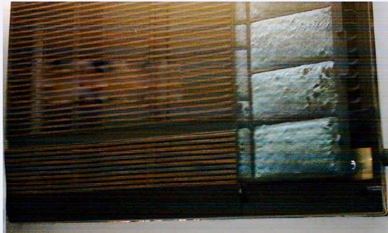
Figure 1. Photograph showing grossly contaminated filter of the Window mounted Air Conditioning unit of the operation theatre
