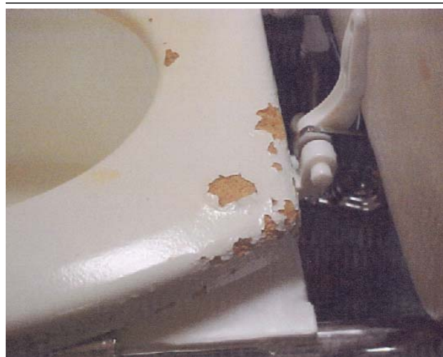
Figure 1: Damaged surfaces impede adequate cleaning
